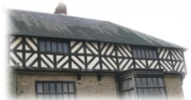
These photos were taken in Mill Street
