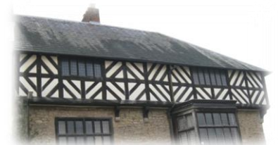
These photos were taken in Mill Street
